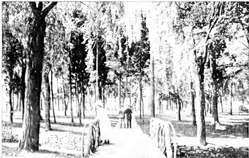
BRIDGE OVER THE SULPHUR STREAM IN THE SANITARIUM PARK
